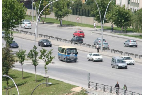
Figure 3. Söğütözü Junction built for motor traffic create risks for pedestrians at urban center
